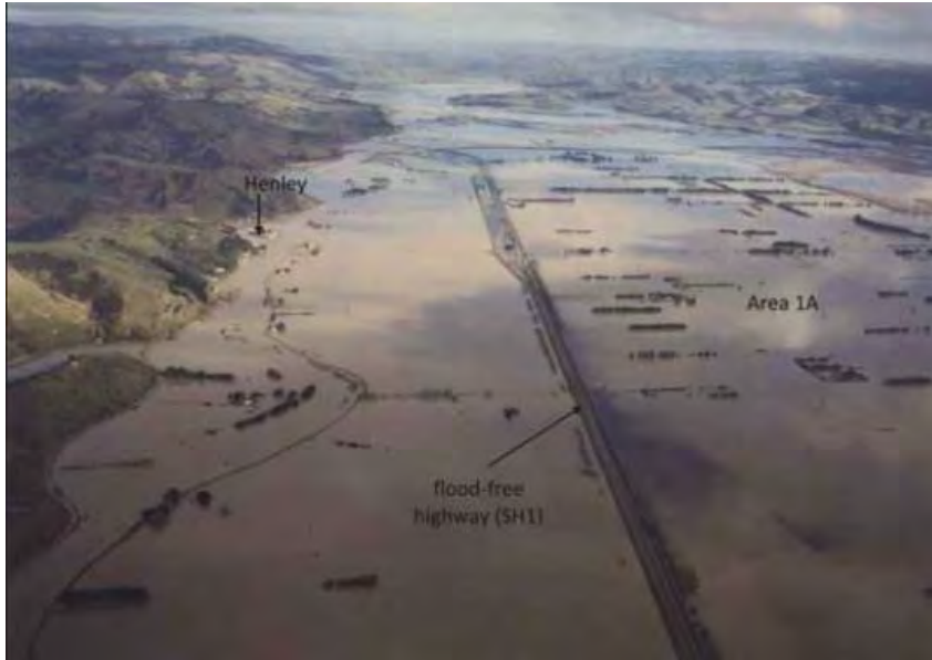
Figure 7-7: Flooding on the West Taieri, following the June 1980 flood event (Goldsmith et al., 2015).
