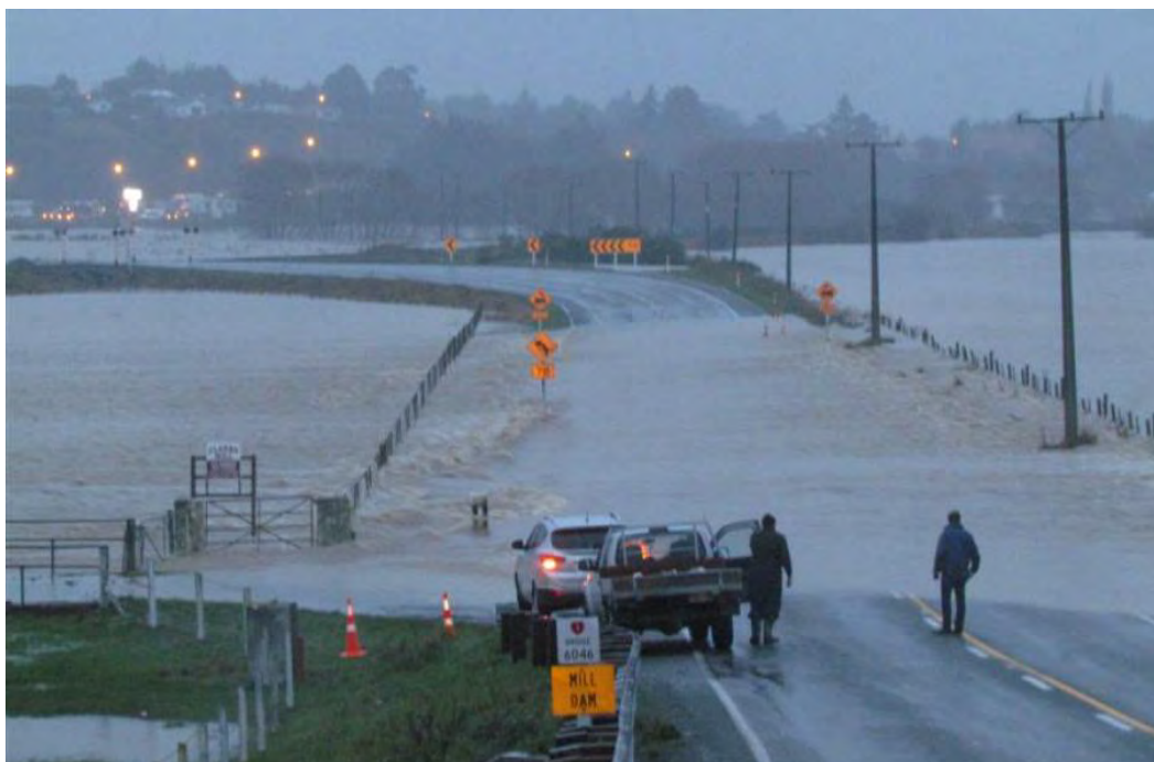
Figure 6-12: Flooding on SH1 at Mill Dam, north of Maheno, Otago in 2013 (Otago Daily Times, 2013).
