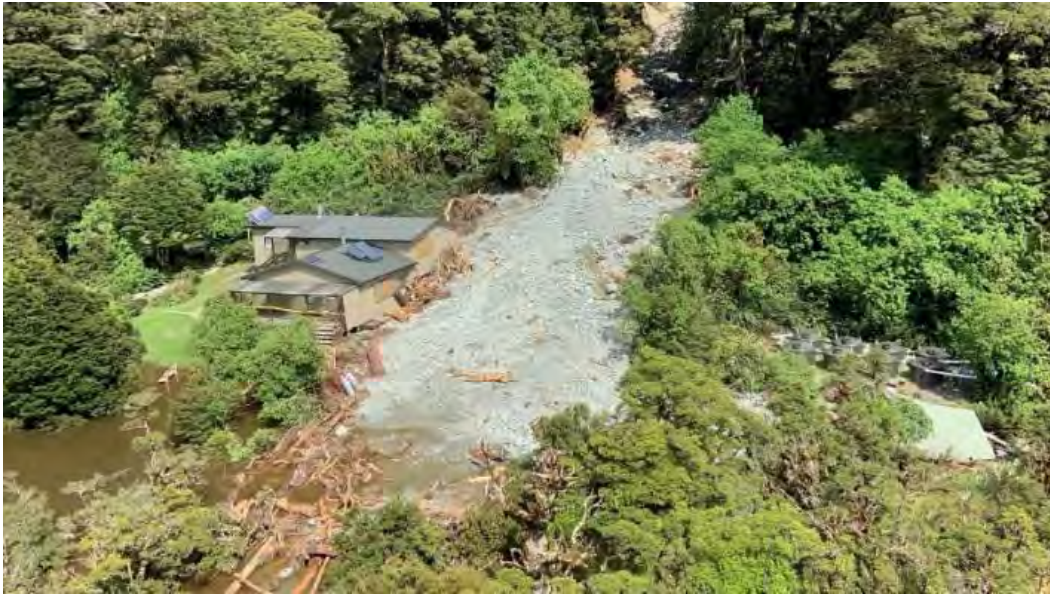
Figure 6-14: Routeburn track hut closures after flooding (Stuff, 2020).
