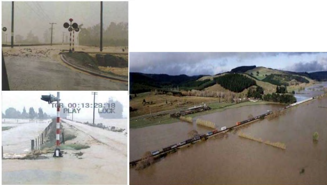
Figure 7-19: Taieri Gorge Railway (left) and South Island Main Trunk (right) inundated by flood waters in the April 2006 floods (Goldsmith et al., 2015; O'Sullivan et al., 2013).
