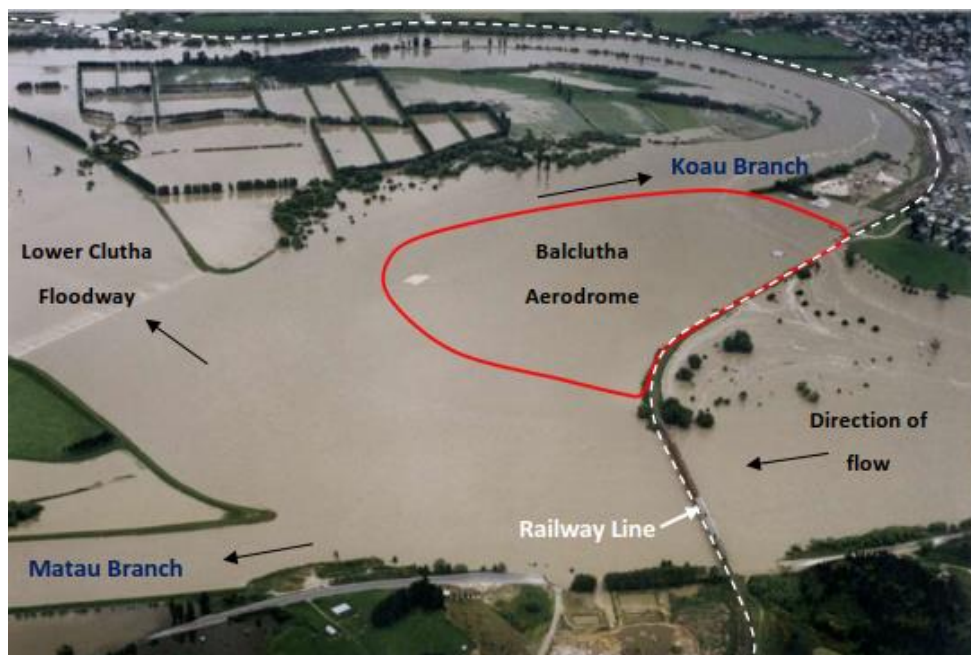
Figure 7-8: South Island Main Trunk railway (white dashed) and Balclutha Aerodrome (red) during the November 1999 flood (Hornblow et al., 2016).
