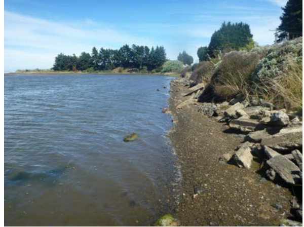
Plate 34: Downstream at Site 9 Kaikorai Lagoon
