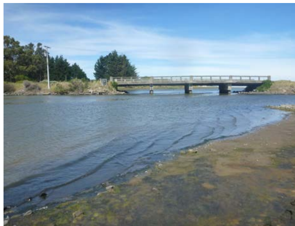
Plate 6: Downstream at Site 2 Kaikorai Lagoon
