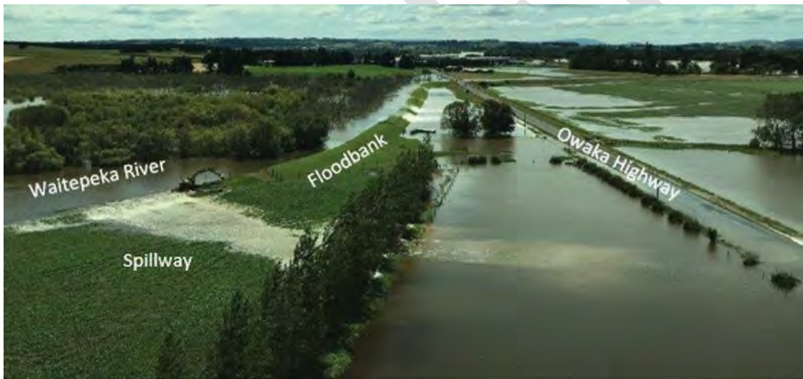
Figure 12 Flood Protection asset, Waitepeka Floodbank during the February 2020 flood event
