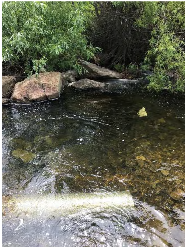
Figure 3: Looking past screened intake towards rock weir outlet
