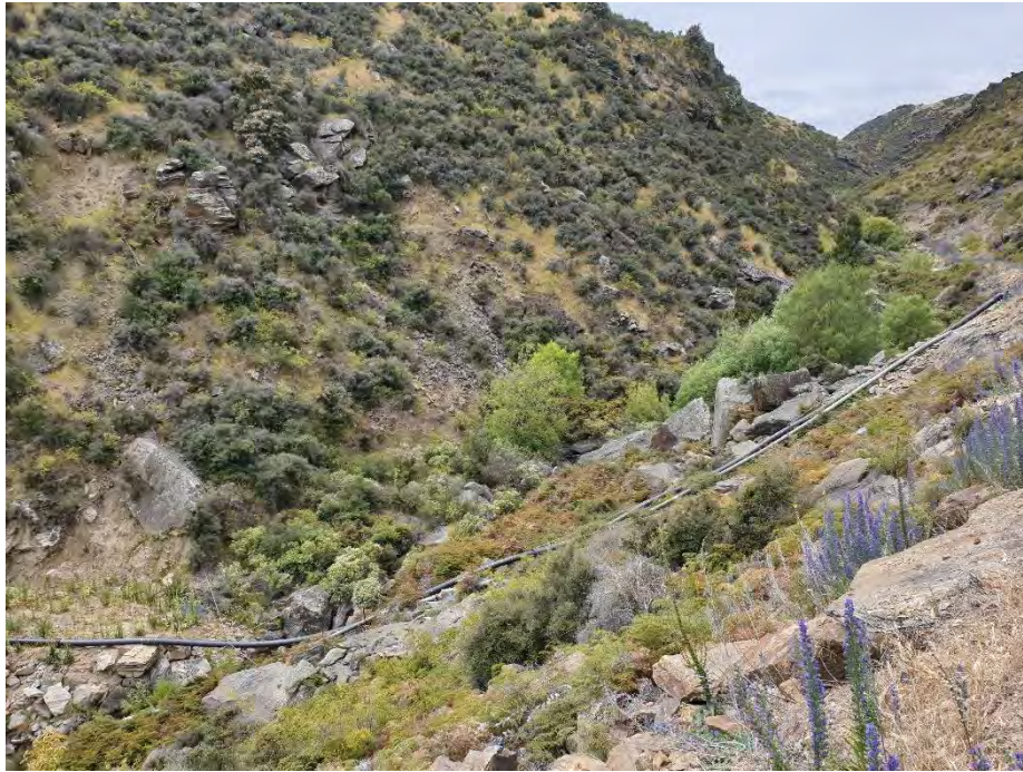
Figure 16: Looking past the applicant's Bendigo Creek pipeline towards the intake
