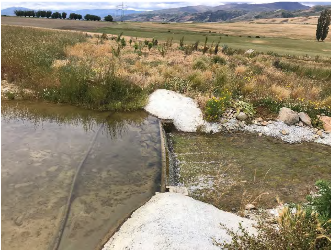
Figure 7: Pond spillway
