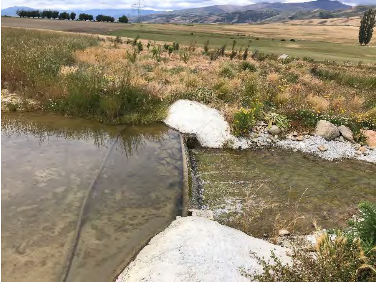
Figure 6: Bendigo Pond spillway and beginning of overflow channel
