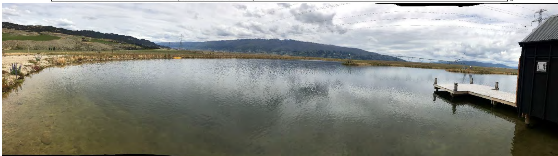
Figure 1 & Figure 2: Bendigo Pond asbuilt and looking west across Bendigo Pond towards crest
