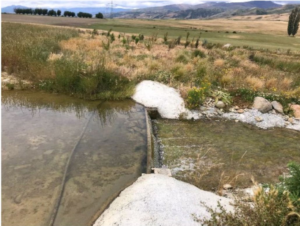
Figure 3: Photograph of operation spillway on Bendigo Station Pond. Source: Application.
