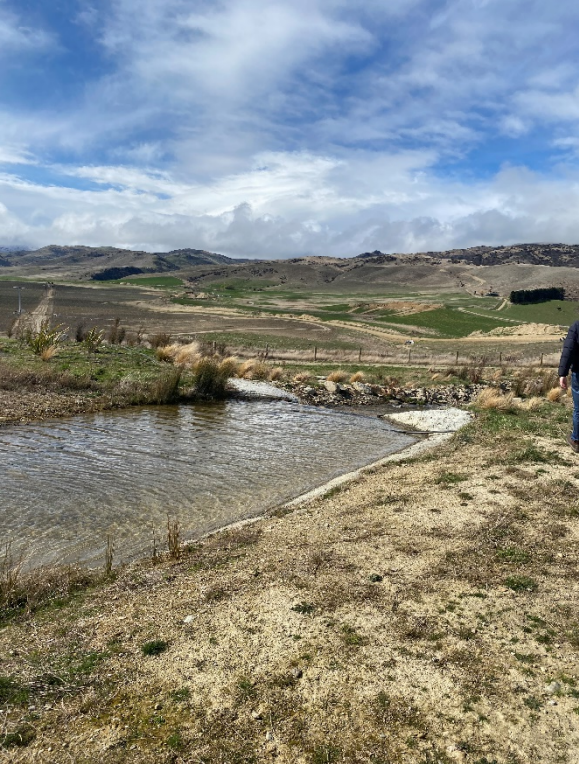
Figure 8: Spillway weir looking downstream
