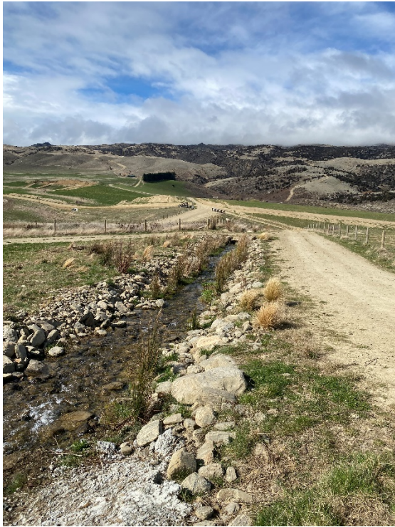
Figure 10: Spillway diversion channel flowing towards Bendigo Creek.
