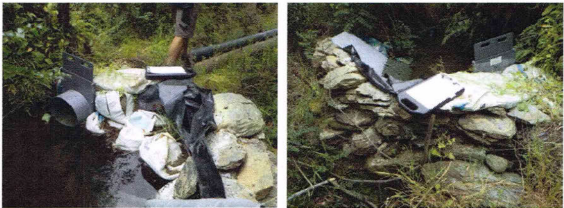
New Chums intake – dammed with a rock wall, bags & plastic.
