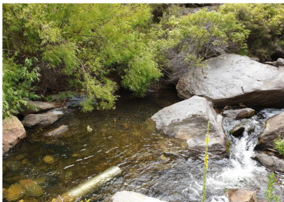
Figure 2: Photograph of intake in Bendigo Creek. Source: Application.
