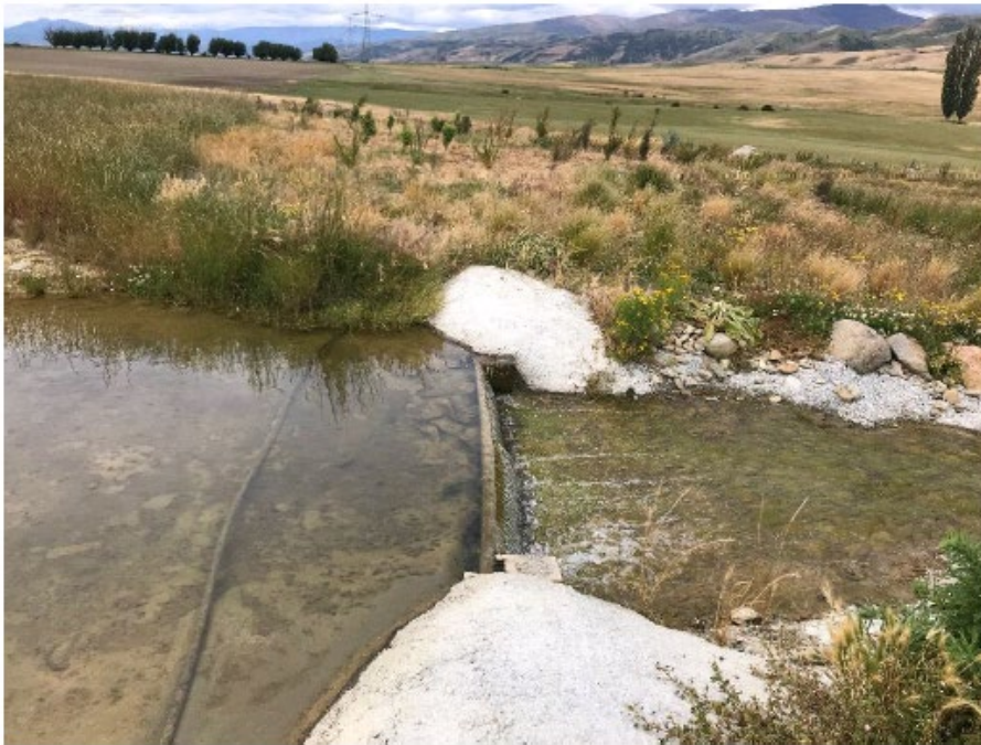
Figure 9: Photograph of operation spillway on Bendigo Station Pond. Source: Application.
