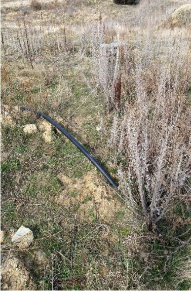
Figure 5: Stock water drinking pipeline. Source: Site visit photo.
