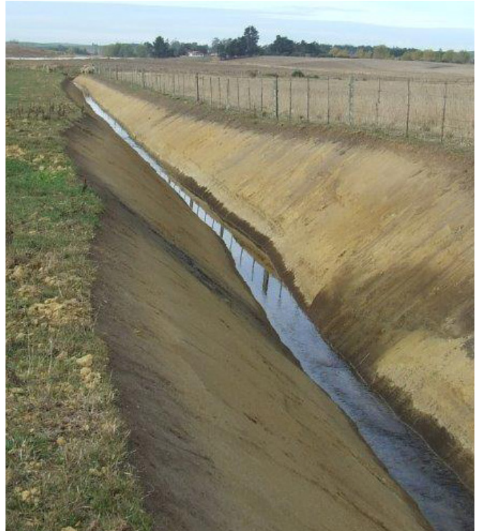
Modified or straightened rivers — while this may look like a drain, it is a river because although it is modified, it has a natural catchment (Friston Stream).
