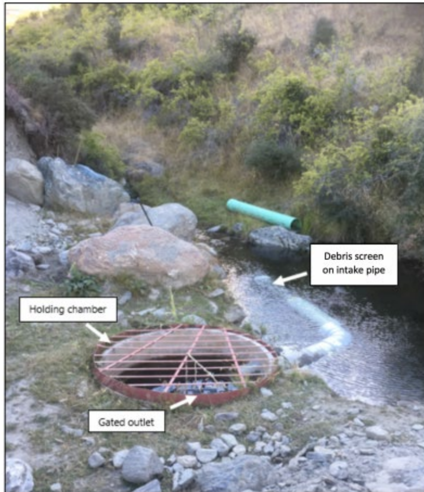
Figure 3: Upper Royal Burn intake showing the holding chamber, gated outlet and ponded area surrounding the intake pipe. Source: Application.
