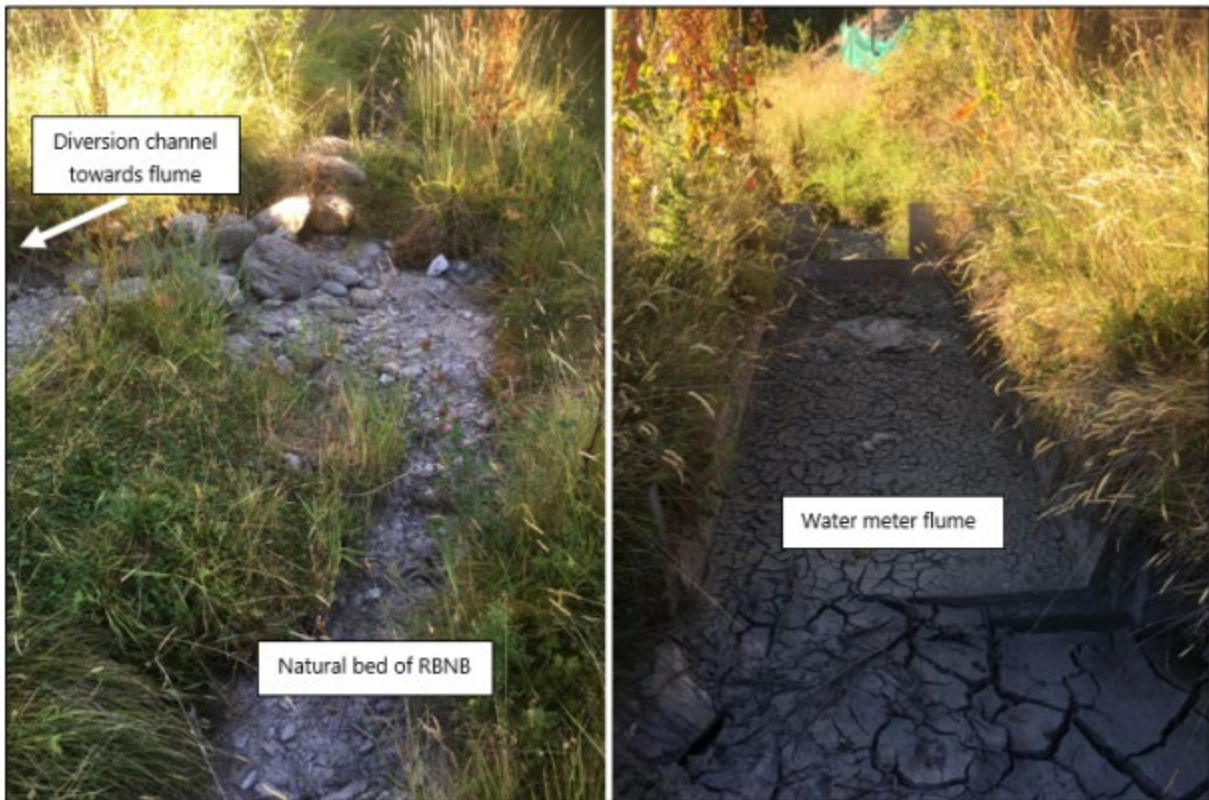
Figure 5: Lower Royal Burn intake showing the natural bed, diversion channel toward flume and the water flume. Source: Application.
