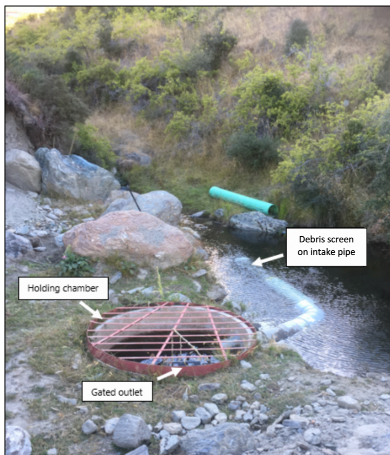
Figure 2: Intake structure at Upper RBNB point of take (RM14.364.01 & 96285)
