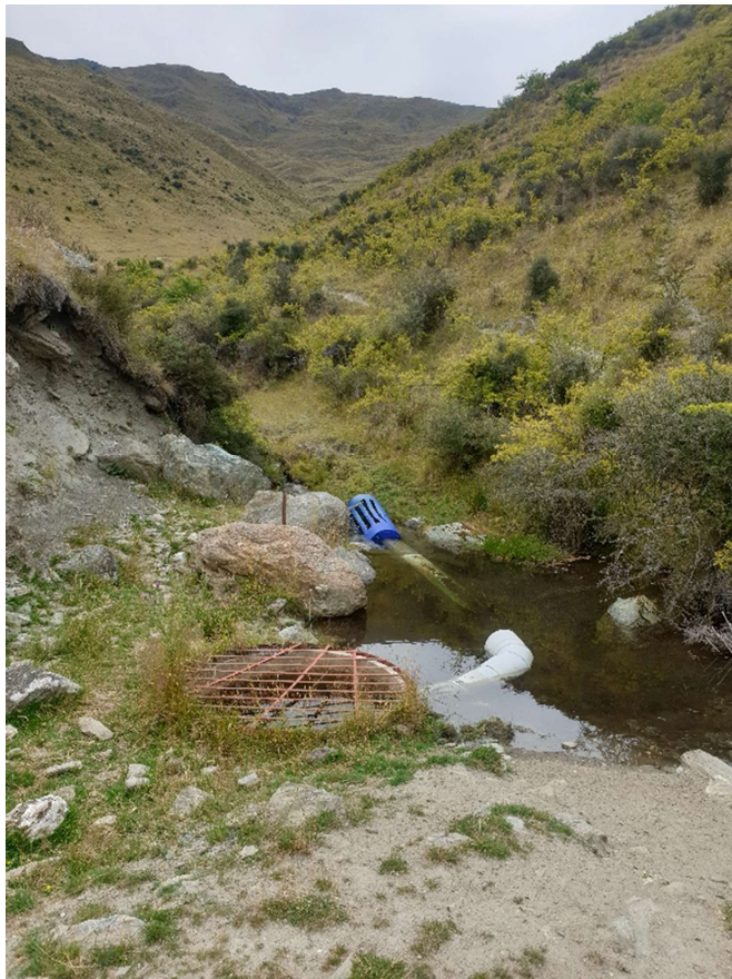
Figure 18: Dam intake
