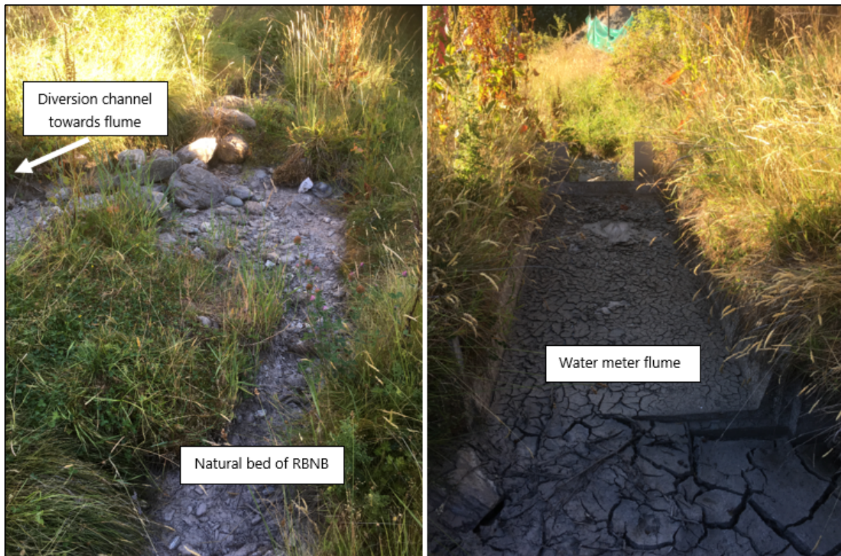
Figure 3: Intake structure at Lower RBNB point of take (97029 & 3037B)
