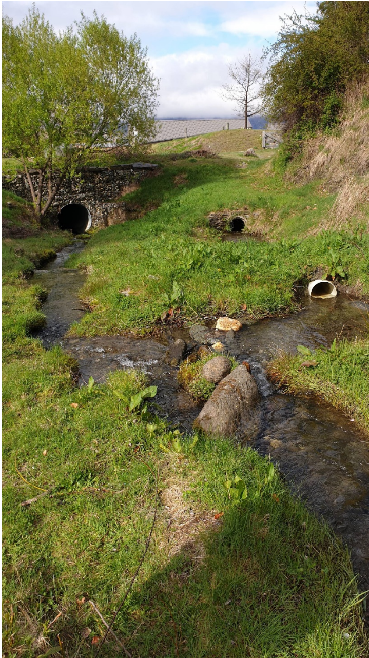
Photograph 12: View looking downstream from above the point that the Royal Burn North Branch flow is split at the Lower take point. Note that there are no flow control devices at all at this take point. Also note that this flow represents 50% of the approximated 50% of the already taken flow at the upper Royal Burn take.
