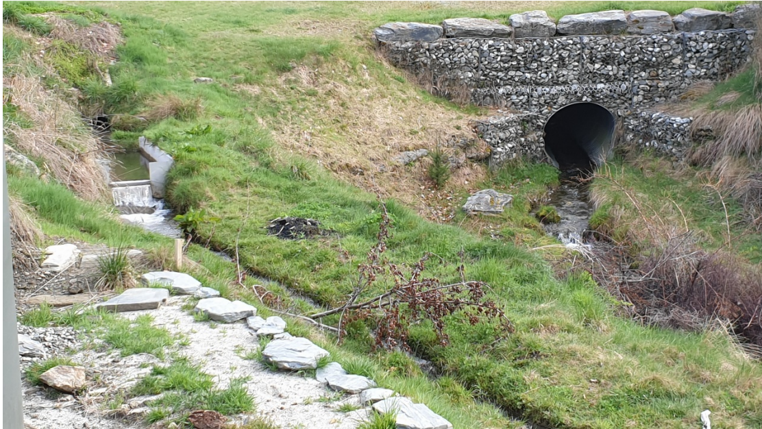
Photograph 10: View of Royal Burn North Branch looking upstream towards the Lower take point, situated slightly upstream from this culvert. Maximum flow depth in culvert was 175 mm. On the left-hand side of photograph is the rectangular weir which measures flow in Brodies Race. On the day (27 th October 2020) the photograph was taken approximately 50% of the flow at this point was going down Brodies Race.
