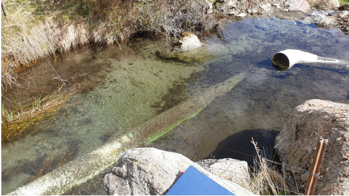
Photograph 6: View looking at intake structure of the Upper Take location on the Royal Burn North Branch. Flow is collected via a large diameter pipe, then flows through a large chamber (to the right of the pipe) before flowing down a pipeline and then either into the storage pond, or down to the central collection point below Glencoe Road. Pipe is less than half submerged, and in chamber (see below) it is fully submerged.
