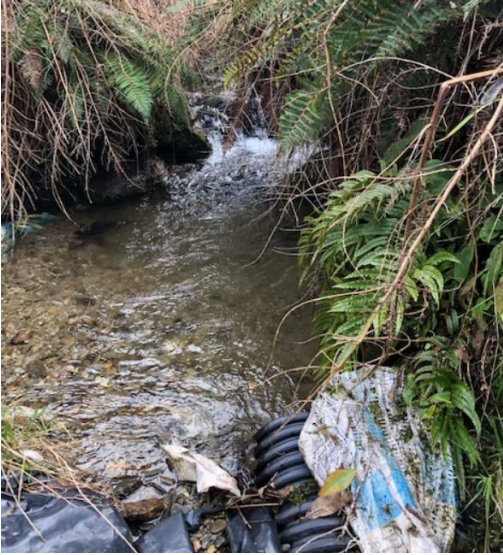
New Chums Creek Water Outtake
