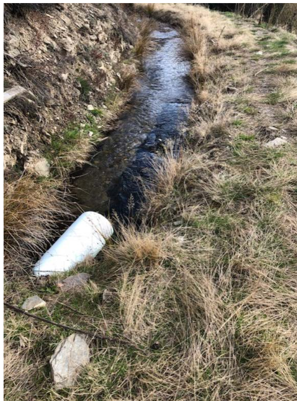
Pipe extraction to the New Chums Historic Mining Raceway
