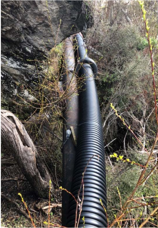
Newly Constructed Pipes
