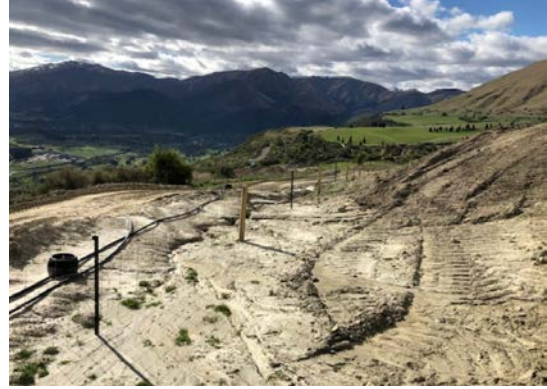
Earth works on escarpment facing North
