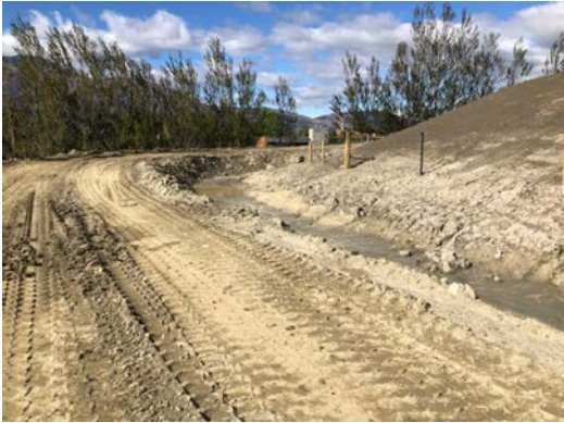
Earth Works with silt wash in small stream
