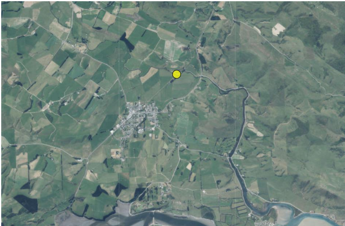
Figure 9. Owaka WWTP and discharge point in relation to Owaka Township and wider environment (Source: Otago Maps)
