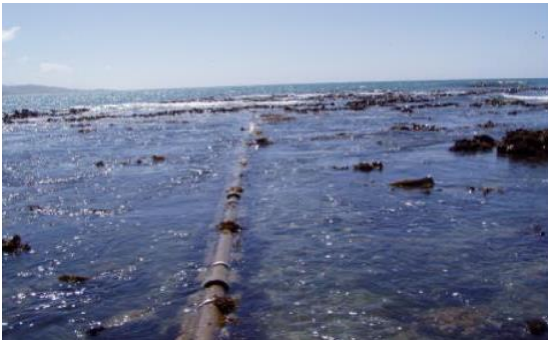
Figure 8. Wastewater pipe leading to the point of discharge (Source: 2008.690)
