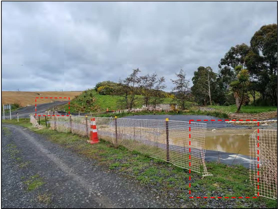
Photograph 3: Orange netting which requires replacement around the northern stormwater detention / sedimentation pond.
