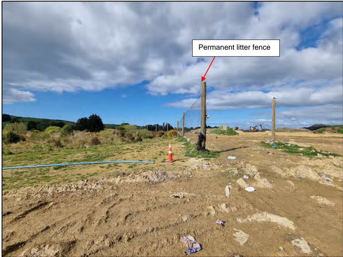
Photograph 9: Current permanent litter fence to be relocated closer to the tip face.
