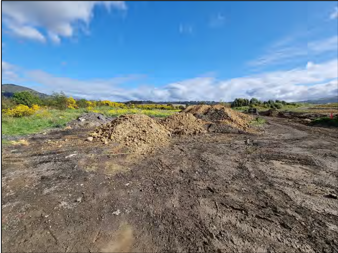
Photograph 5: Stockpiled clay material adjacent to the current asbestos disposal area to be used as capping material.
