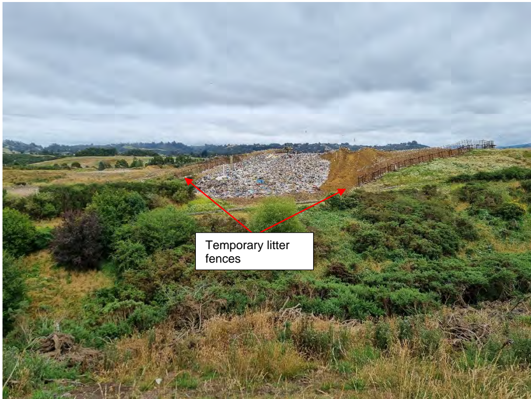
Photograph 5: View of the current tip face, indicating the location of the temporary litter fences looking north.
