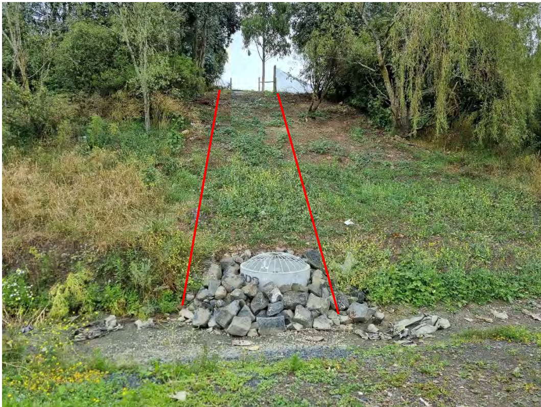
Photograph 14: New culvert has been installed adjacent to the green waste disposal area, looking south west.
