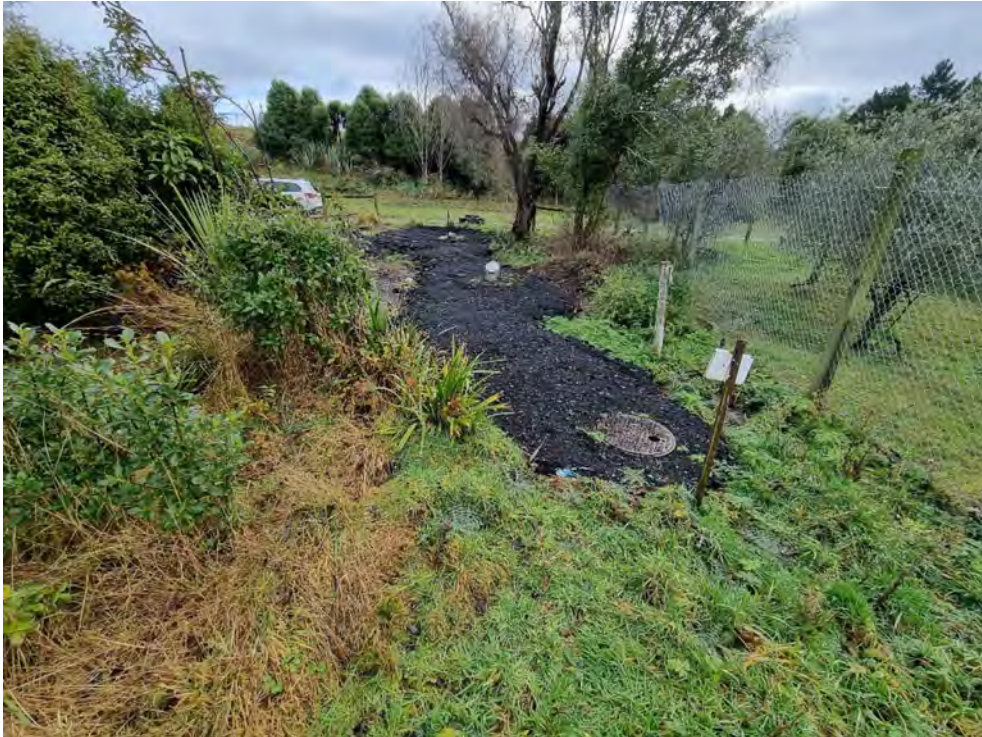
Photograph 19: Crushed asphalt has been lain along well line 8 to stabilize the concrete well plinths.
