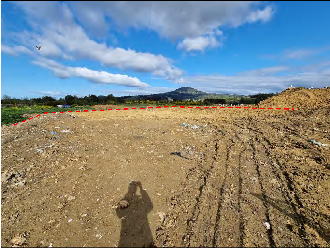
Photograph 13: Intermediate cap over an area to the west of the current tip face.
