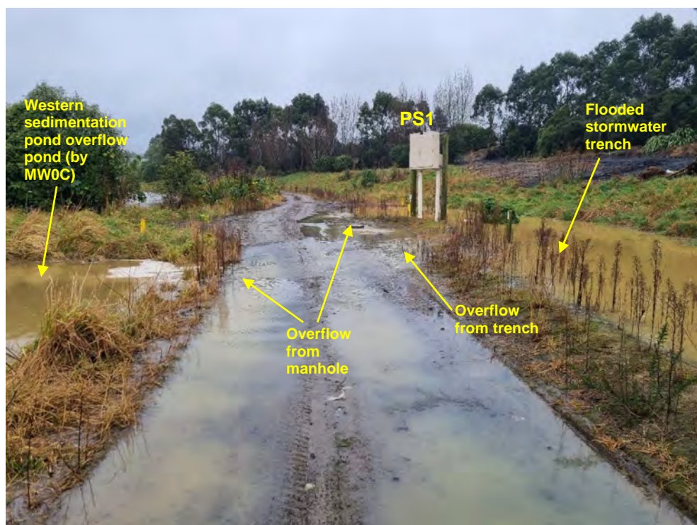
Photograph 6: Flooding of the leachate channel and overflow from PS1 into the W pond (by MW0C), looking north.
