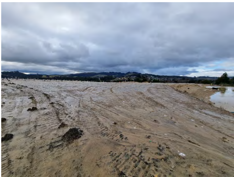
Photograph 18: Recently placed capping material over the northern portion of the landfill, looking north.
