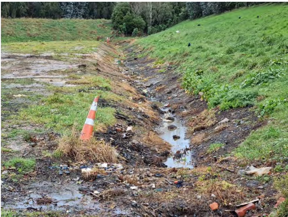
Photograph 4: Moderate volume of waste materials present in the stormwater channel along the south west boundary of the compost area.
