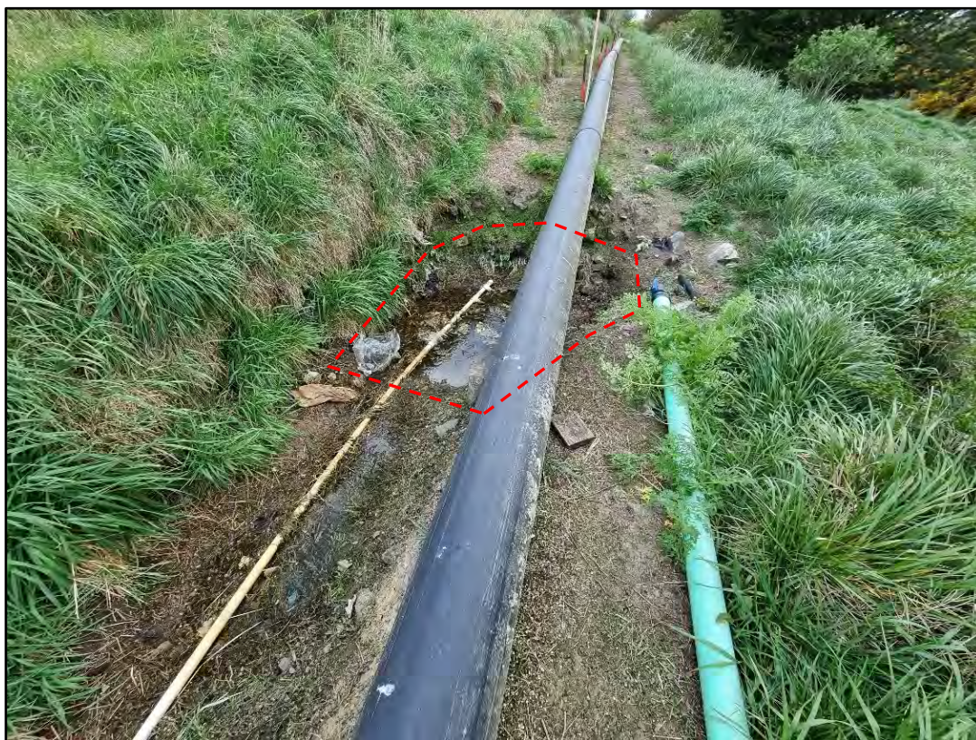
Photograph 1: A slight hole is present in the ground surface beneath the gas line to the east of line MW0.
