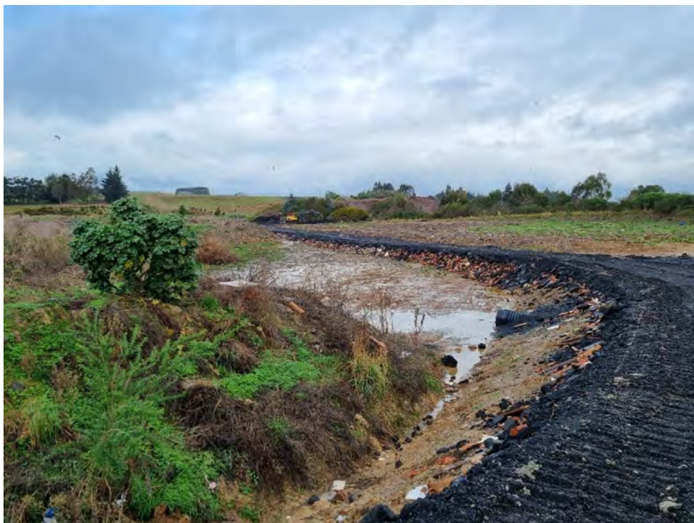
Photograph 14: New access road constructed of demolition materials (brick) and crushed asphalt.
