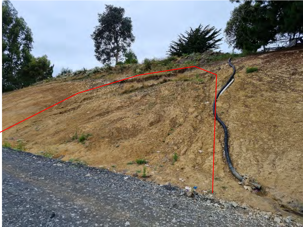
Photograph 7: Area of minor slump / erosion on the constructed road to the borrow pit.
