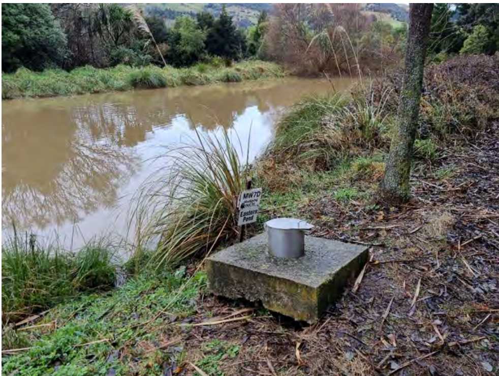
Photograph 20: Well MW7D's concrete base has been undercut and is unstable.
