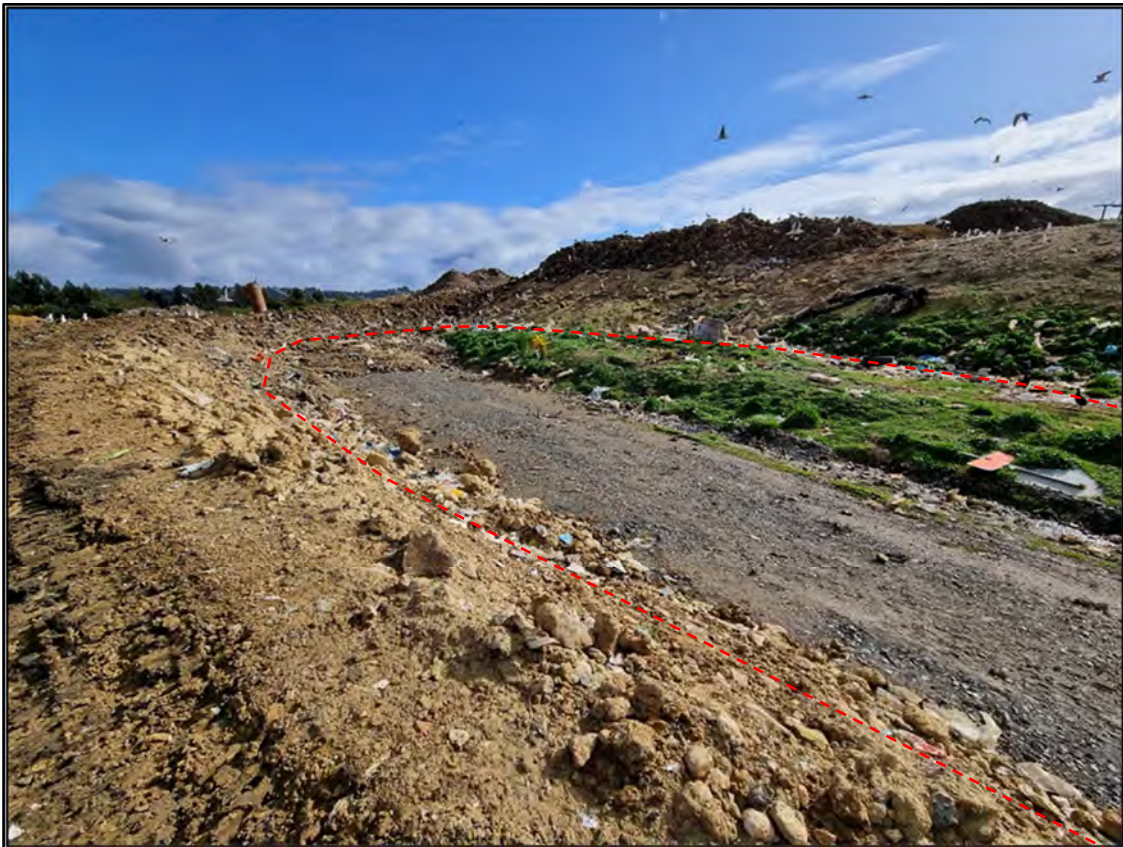
Photograph 14: Area prepared to receive asbestos materials to the west of the current tip face.
