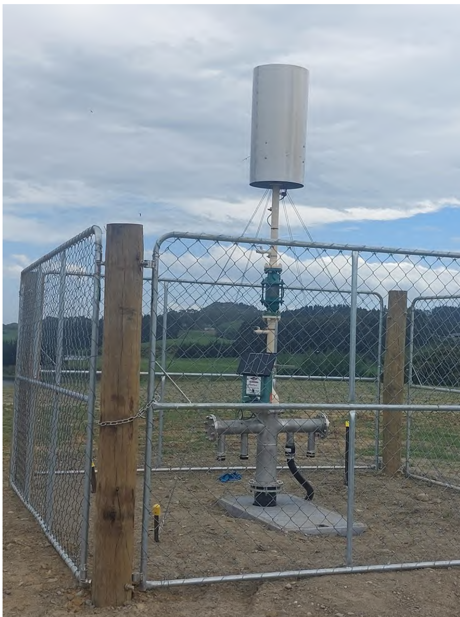
Figure 2.2: Solar Spark® candlestick style LFG flare fitted with a stainless steel visibility shield (shroud) installed at the Eastern Landfill (source WMNZ).
